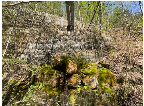
Splash pad and tensioned bulging wwm. Wicking socks visible.
