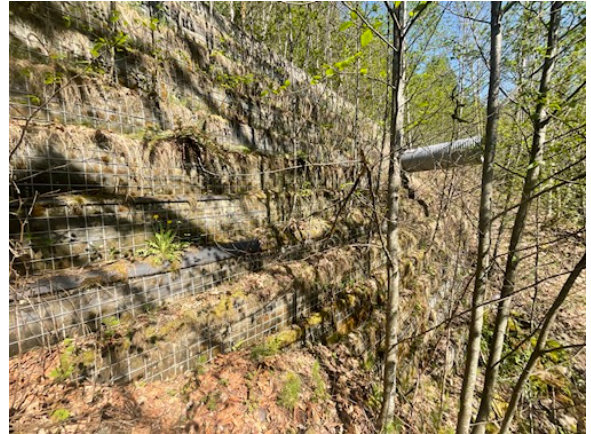
Wall facing. wwm tensioned up but not yielded.
