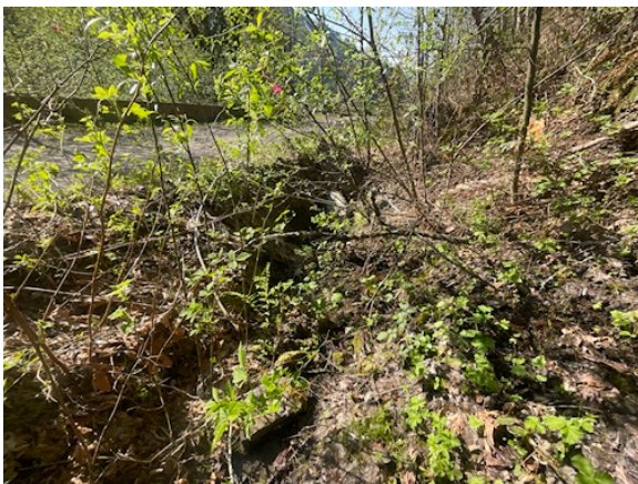
Culvert inlet brushy but functional
